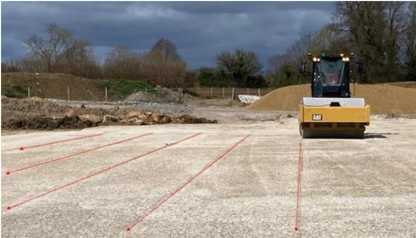
Figure 22 - Semi-Autonomous Compaction showing aligned passes with
