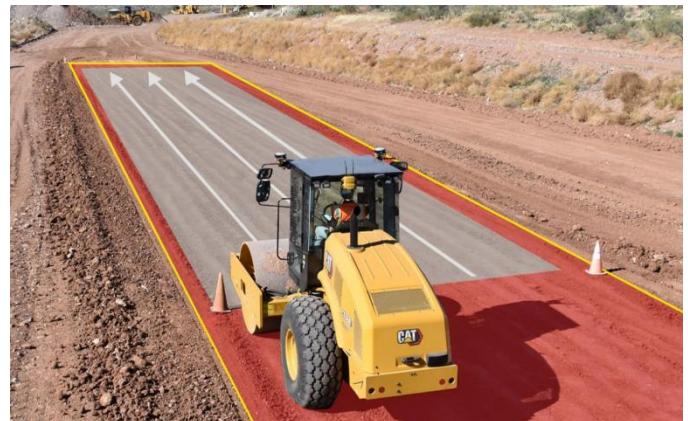
Figure 19 - Example of compactor trial site
