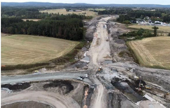
Figure 17 - Example project existing aerial view xli
