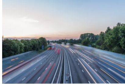
RDP & Smart Motorway Alliance
